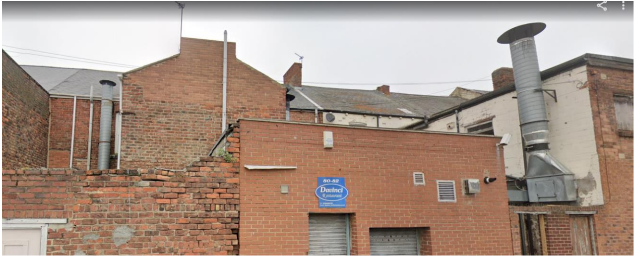
Kitchen Extraction Located on Southern Façade of Food Establishments
